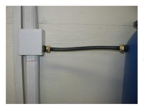
7. Connect diverter to your rain barrel using the provided hose.
