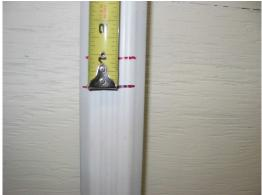
5. Cut a triangular piece about 1 inch tall from one side of the downspout.
