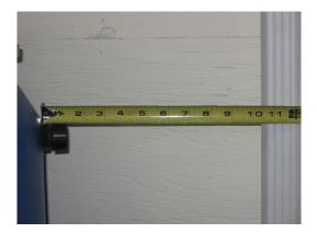
3. Measure across from overflow (top) fitting on rain barrel when it is at installed height and mark downspout at same level.
