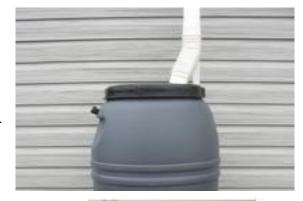
2. Another option for installation is the use of a diverter hose. Only part of the water is directed into the rain barrel, with the rest going down the downspout. It takes about an hour for this type of installation to fill a rain barrel, and after the barrel is full, the water directs itself through the downspout, eliminating the need for an overflow hose.
